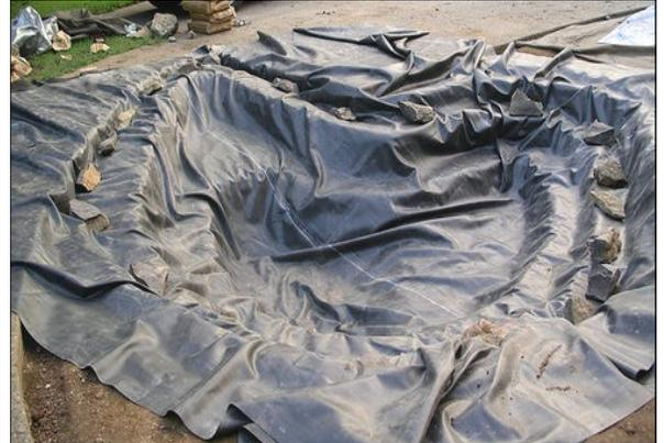
A pond liner installed showing shelves in the pond for different types of plants.
